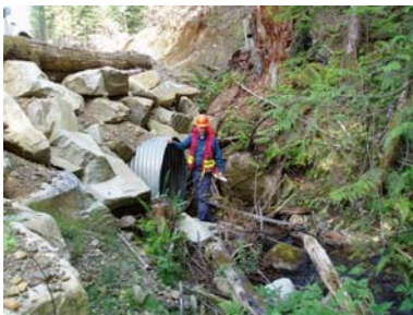
Shawn Hamilton inspecting a corrugated metal stream culvert at coastal site
