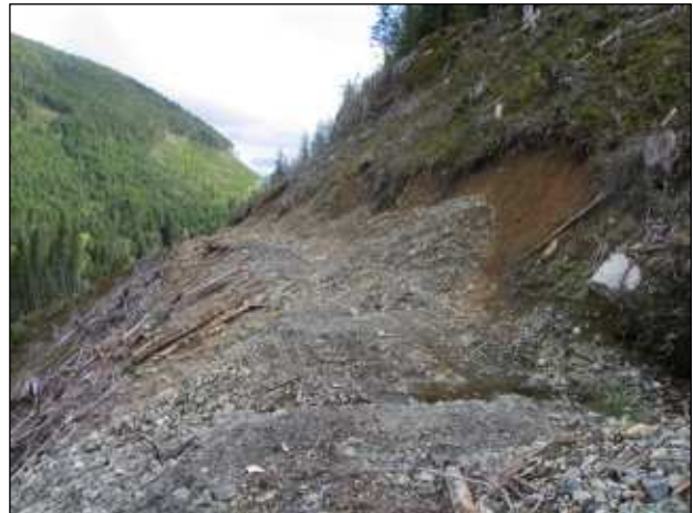
4. Effective pullback and cross-ditch on deactivated road.
